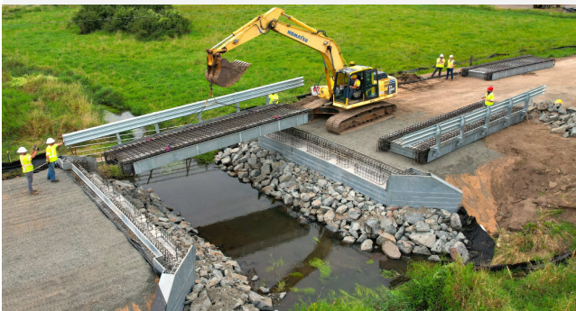
3. Lift InQuik Superstructure Panels onto abutments and connect splice bars.
