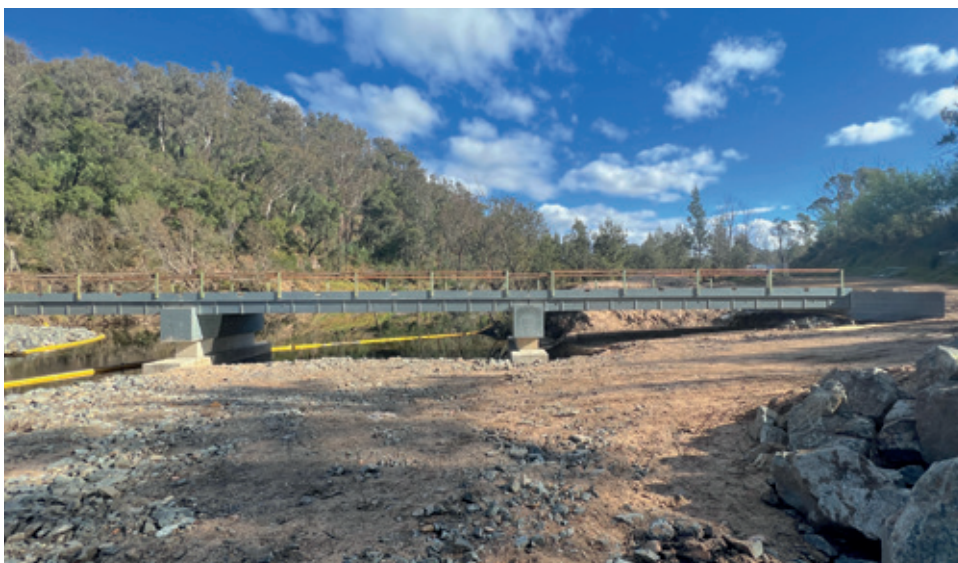
Figure 38. A completed InQuik bridge installation before concrete is poured.
