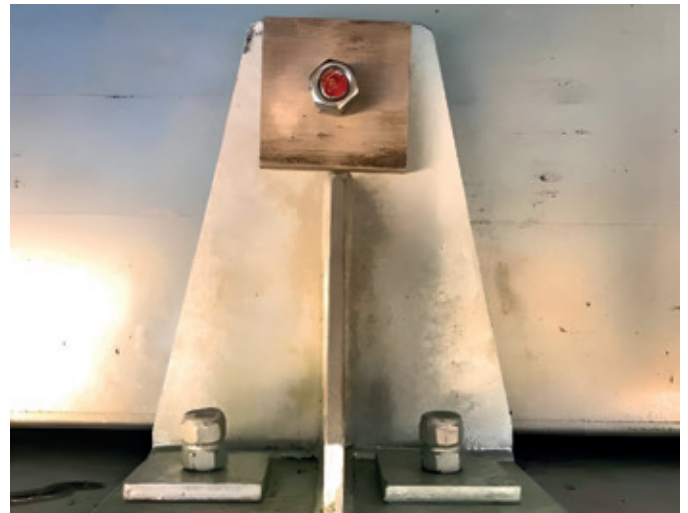
Figure 36. A complete installation of a tie down bracket connecting the deck panel and the pier cap.
