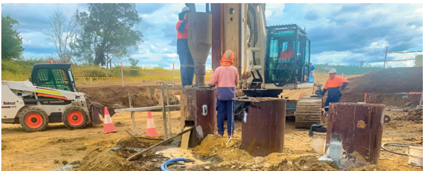
Figure 8. Concrete pipe encasements are used to achieve the required level before the pier cap is installed on top.
