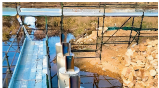
Figure 16. Safety rails and platform erected on one side of the piles.
