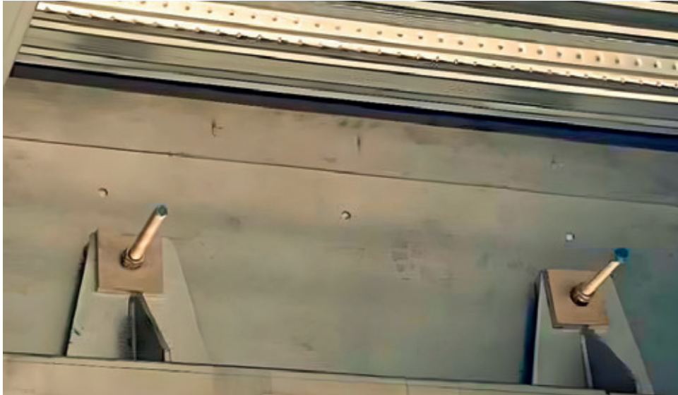
Figure 34. Tie down brackets are used to secure the deck to the pier cap.
