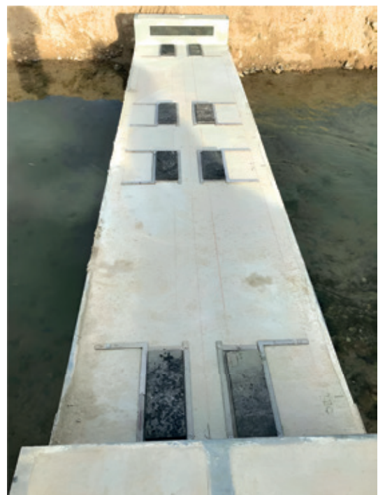
Figure 29. Bearing pads are installed onto the pier cap.
