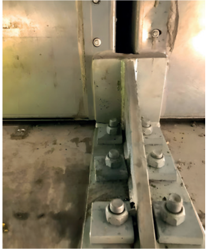
Figure 37. A buffer bracket is bolted into the pier cap, next to the intersection of two deck spans.
