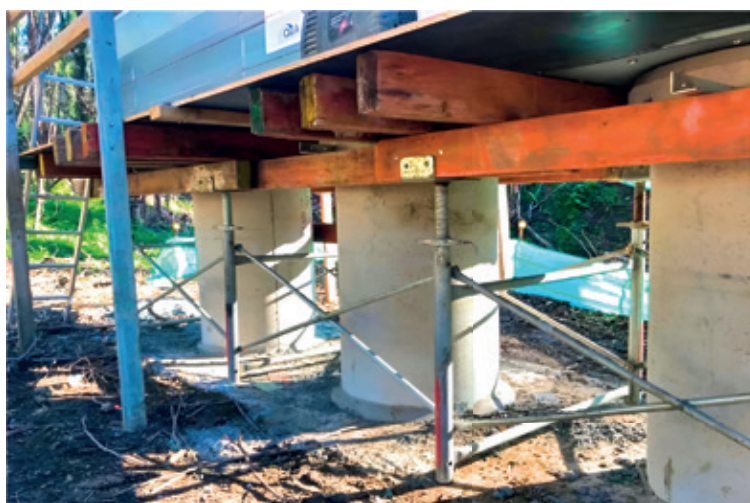
Figure 5. A close-up view of the formwork frame at one of the piles below the pier cap.
