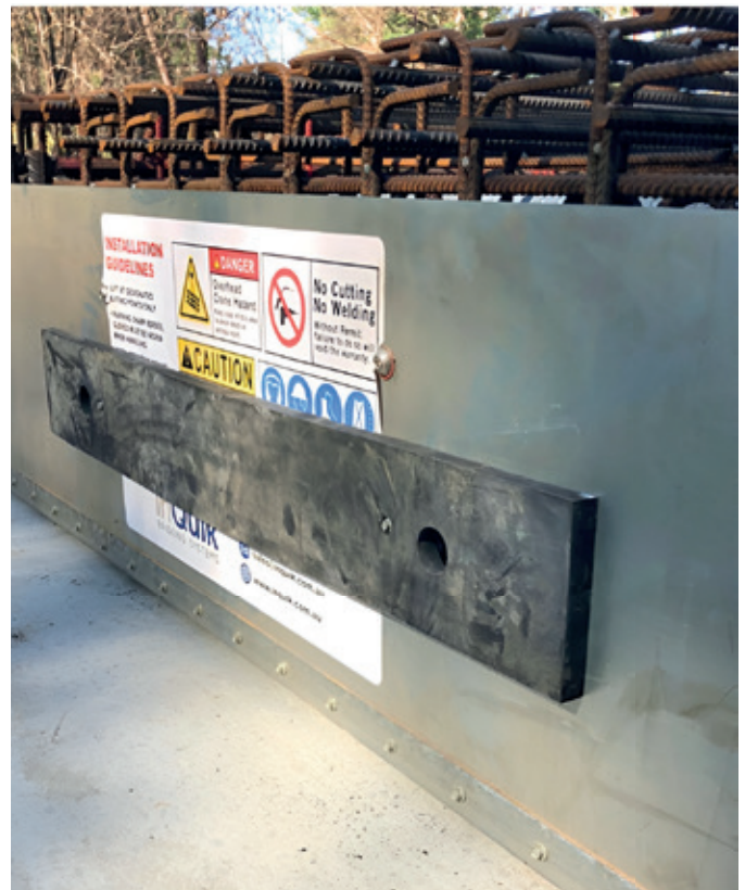
Figure 31. Bearing pads are installed at the end of the deck spans before the next span is installed.
