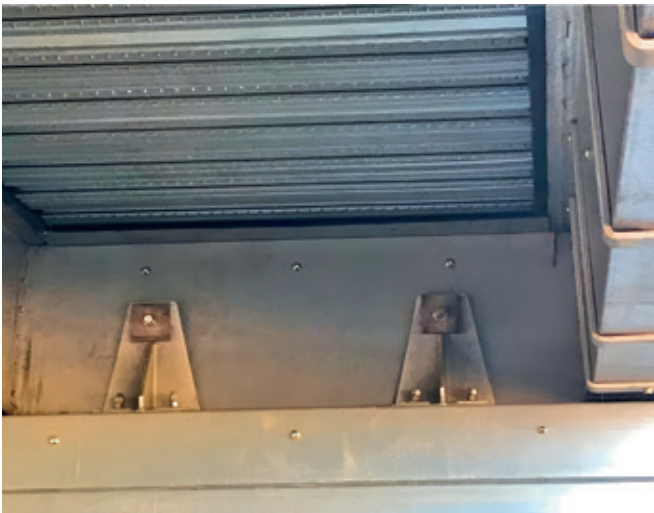
Figure 35. Tie-down brackets connect the deck panel and the pier cap.
