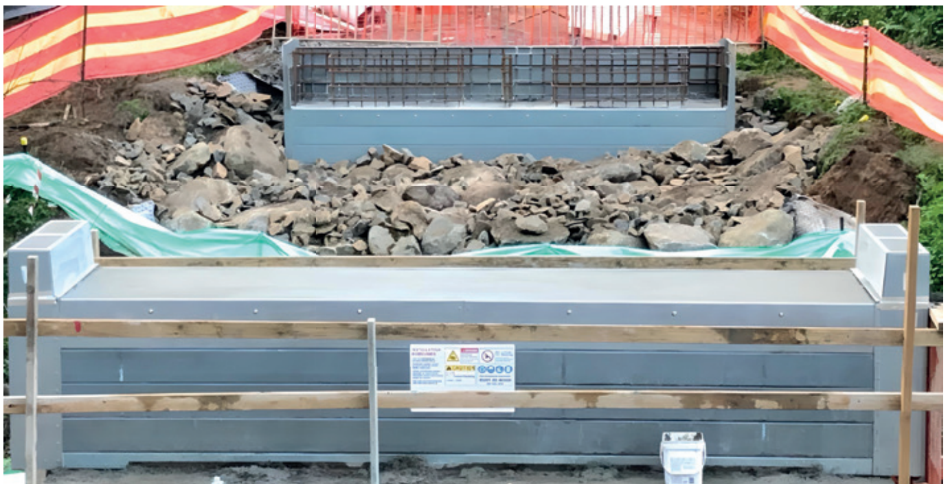
Figure 24. The concrete cures before the deck panels are installed.
