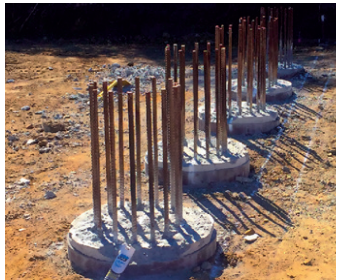
Figure 7. Piles are cured and ready for pier cap installation.
