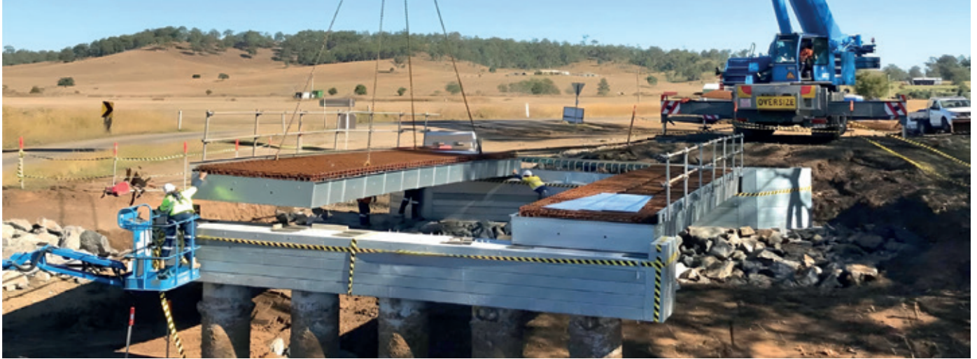
Figure 30. Deck panels are lowered onto the pier cap.
