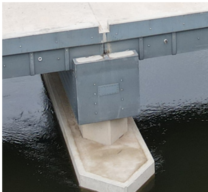
Figure 22. A wash-out hole is included on the side of the pier cap. A small patch up plate is used to cover the hole before the next concrete pour.
