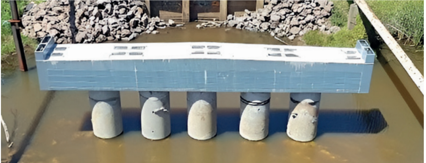
Figure 3. Pier cap installed on top of concrete encased H-piles.
