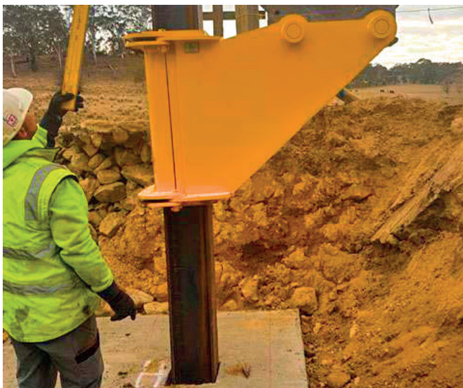
Figure 6. H-pile is driven into the concrete on-site
