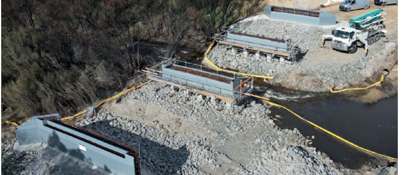
Figure 19. The pier cap must be installed with appropriate scaffolding.
