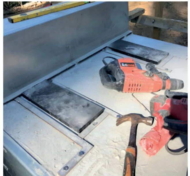
Figure 26. The bearings and retainer strips are installed on the pier cap.
