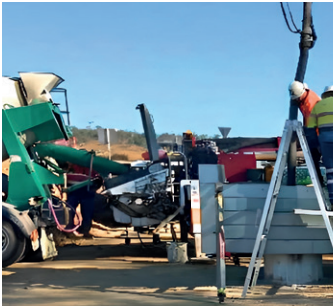
Figure 21. The pier cap is placed on top of the piles before concrete is poured.
