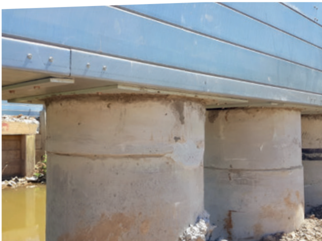
Figure 13. A pier cap placed on top of piles.
