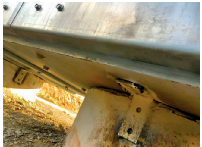
Figure 14. Pier cap support plates and brackets are welded to the steel casing on the piles.
