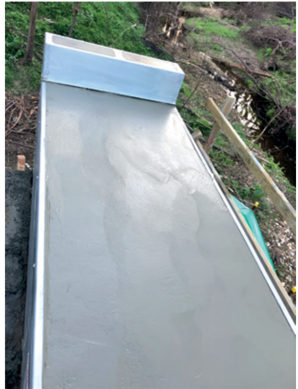
Figure 23. The surface is screeded after the second concrete pour, and the restraint blocks on the pier cap sides are filled with concrete and levelled.
