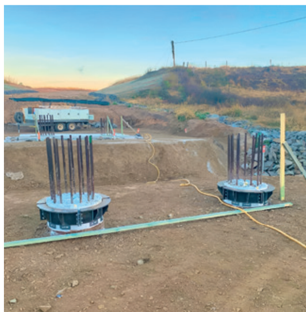
Figure 11. An example of a pile collar placed on top of the concrete pipe encasement.
