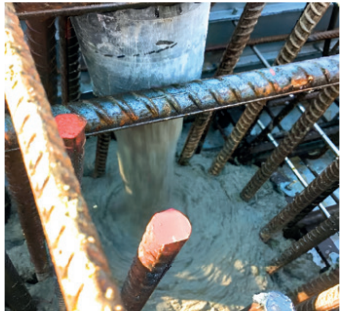
Figure 21. The pier cap is placed on top of the piles before concrete is poured.
