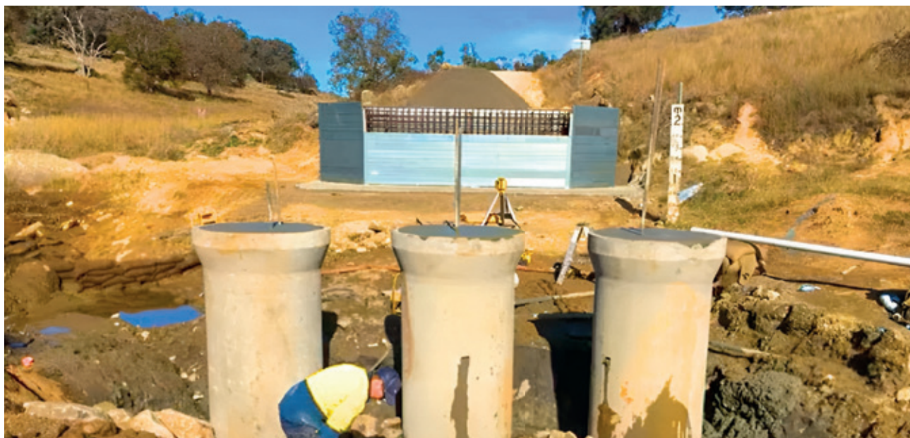
Figure 9. The piles are cured, and the pier cap can be installed.
