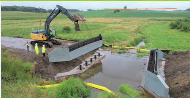
2. Lift InQuik abutments onto foundation and place ready-mix concrete.
