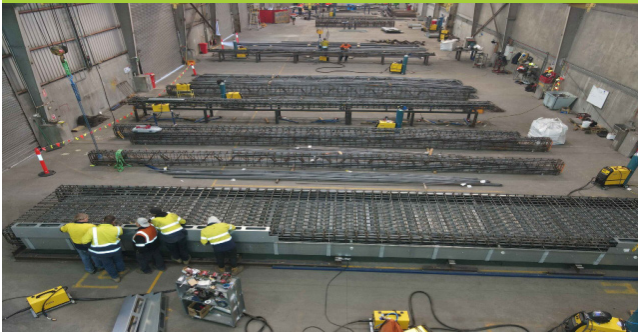
1. Modular components (abutments & superstructure) are prefabricated off-site.
