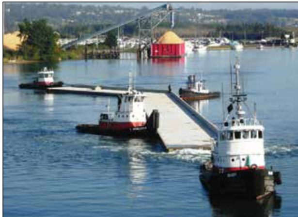
Floating Marina Breakwater, Port Orchard, WA Floating breakwater 100 ksi corner reinforcement. Constructed 2006
