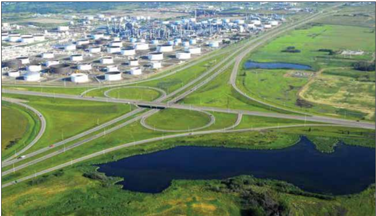
Anthony Henday Drive Ring Road - Edmonton, AB, CAN ChromX rebar used for girders, abutment for 47 bridges. Completed 2013
