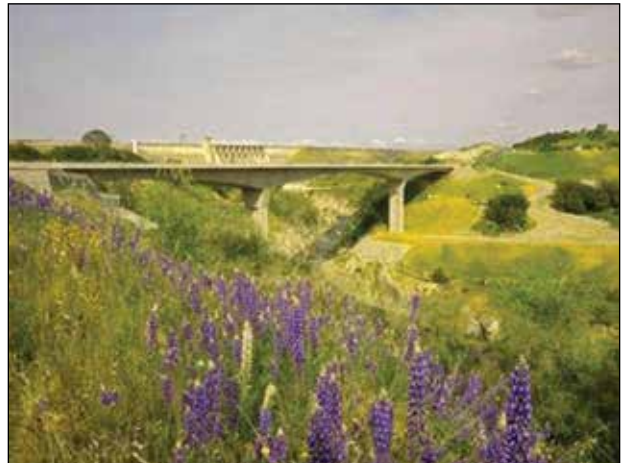
Light Rail Bridge over Alder Creek - Folsom, CA Bridge – ChromX used in abutments, columns and girder (100 ksi design). Constructed 2004
