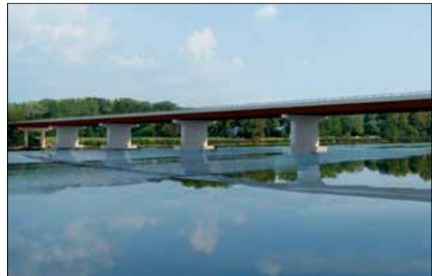
Huguenot Bridge (SR 147) over James River - Richmond, VA Bridge deck was built with ChromX. Completed 2013
