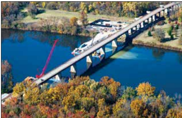
Huguenot Bridge (SR 147) over James River - Richmond, VA Bridge deck was built with ChromX. Completed 2013
