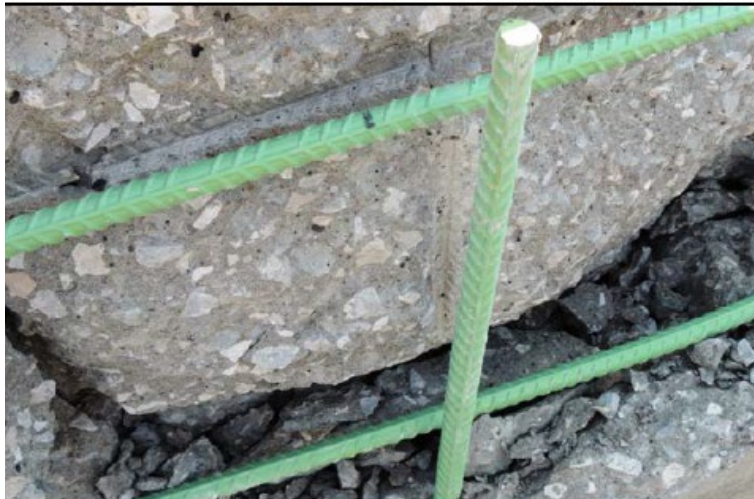
Figure 30 Lack of Bond Between Epoxy-Coated Bars and Concrete Under Impact Loading 11
